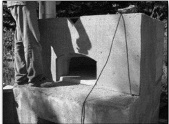
10.4. Attach concrete board.
