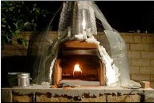
9.3. Rebar and lathe shape the Igloo.
