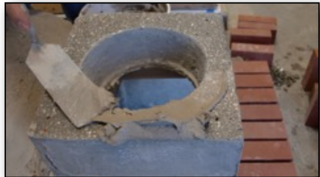
6.4. Apply a bead of refractory mortar.
