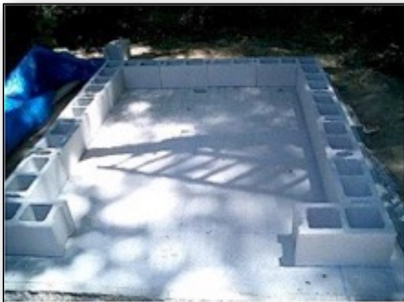
2.1. Carefully lay out the first course of blocks.
