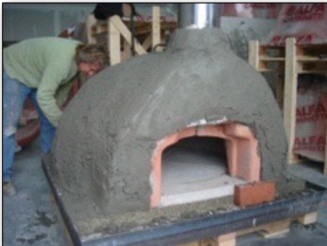
9.4. Rough coat of stucco on wire lathe.
