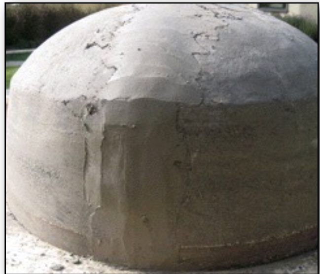
5.2. Seal the outside of the oven dome joints.
