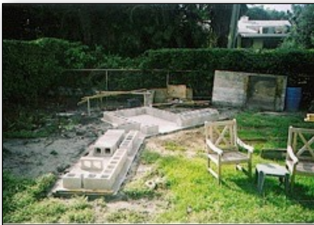
1.4 The foundation and first course of stand blocks.
