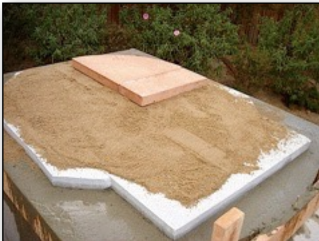
4.1. Set the cooking floor on a thin bed of sand.
