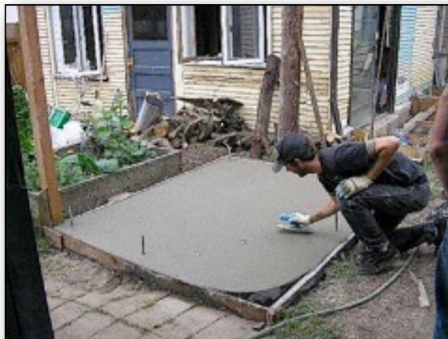
1.2. The finished foundation ready to cure.
