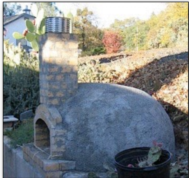
9.2 The oven dome and lathe shape the Igloo.
