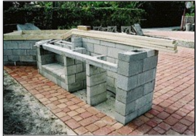
2.5. Stand with cast lintels.
