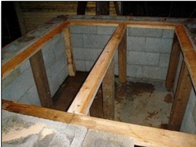
3.1. The form bottom ready for the Hardibacker.
