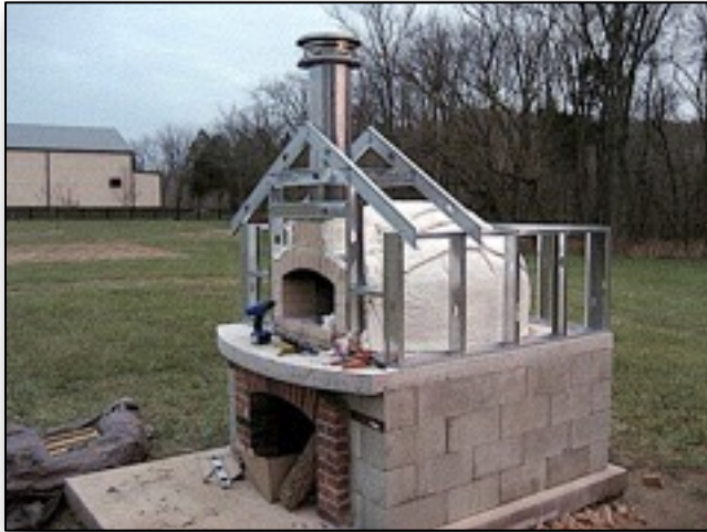
10.3. Metal studs and a gabled roof.
