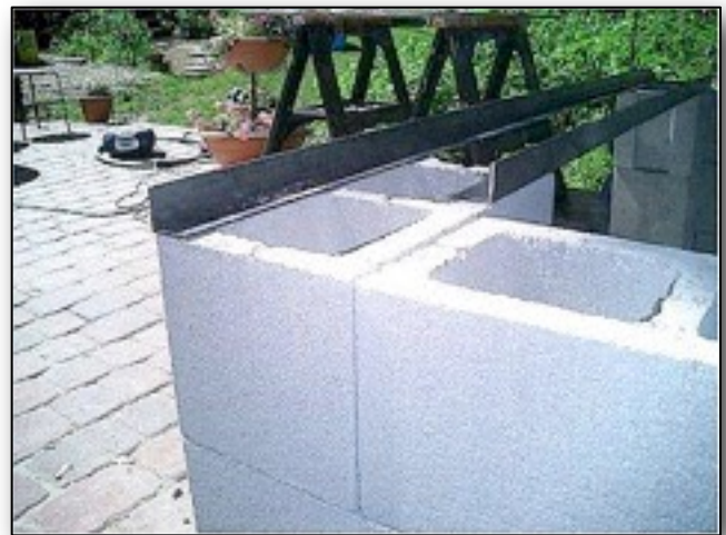
2.2. Cut the back angle iron to leave room for blocks.
