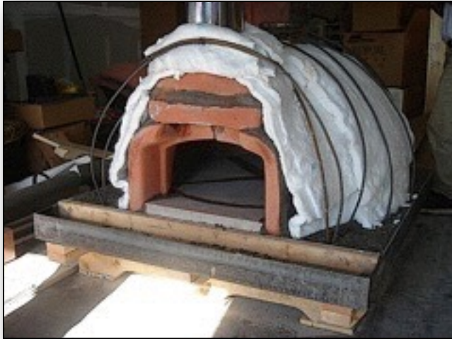
7.1. FB Blanket inside a rebar Igloo frame.
