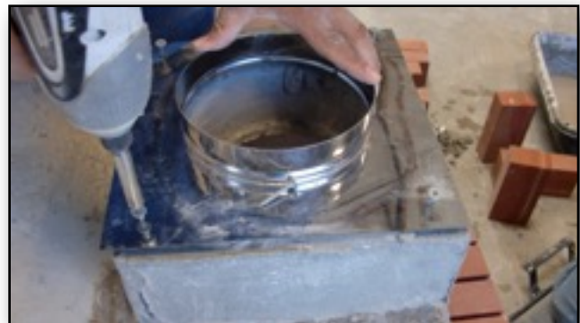
6.5. Screw the anchor plate in place.
