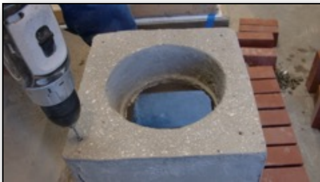
6.3. Pre-drill 5/32" holes to line up with the anchor plate.
