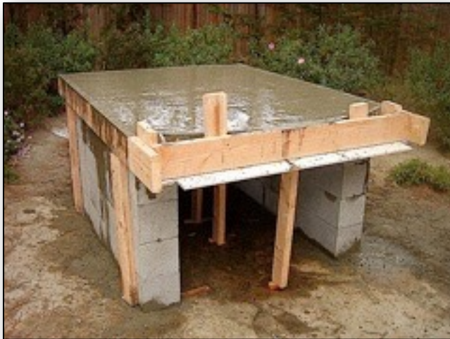
3.6. Structural layer waiting on insulating layer.
