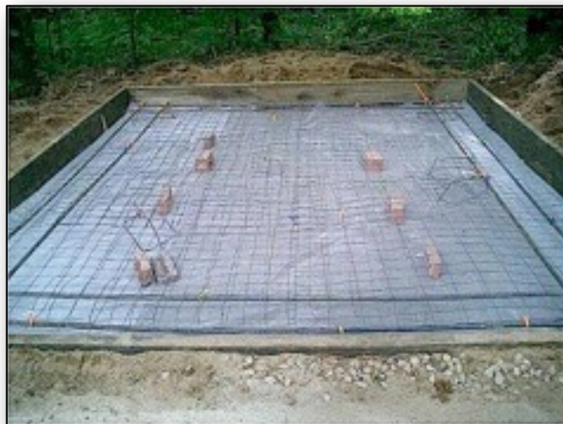
1.1. Framed, lined, with wire mesh and rebar.
