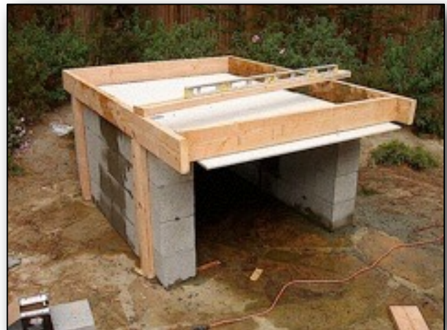
3.3. Hardibacker and form set in place.
