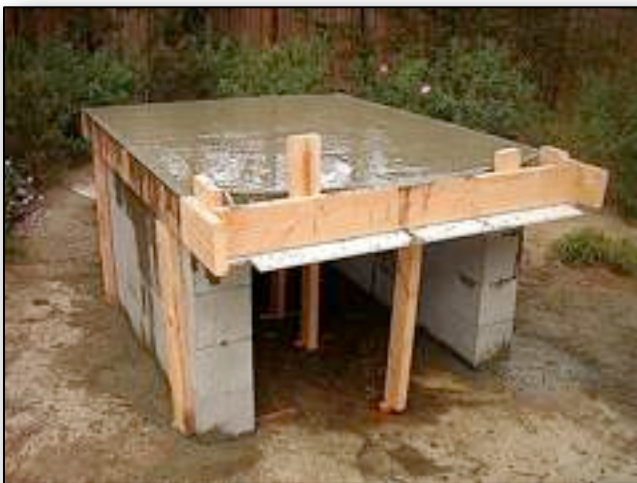
3.6. Structural layer waiting on insulating layer.
