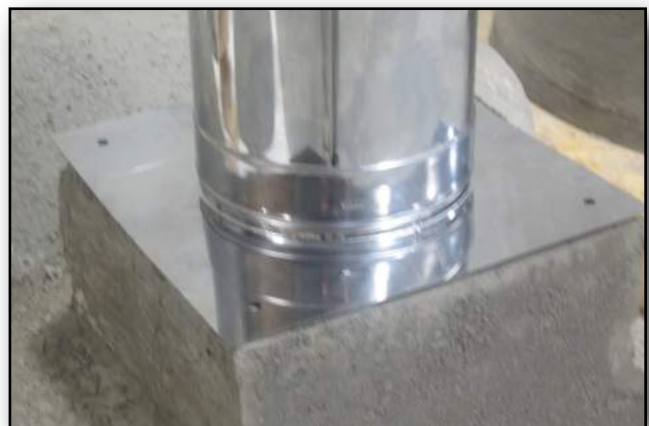
6.3. Attach the anchor plate using concrete screws.
