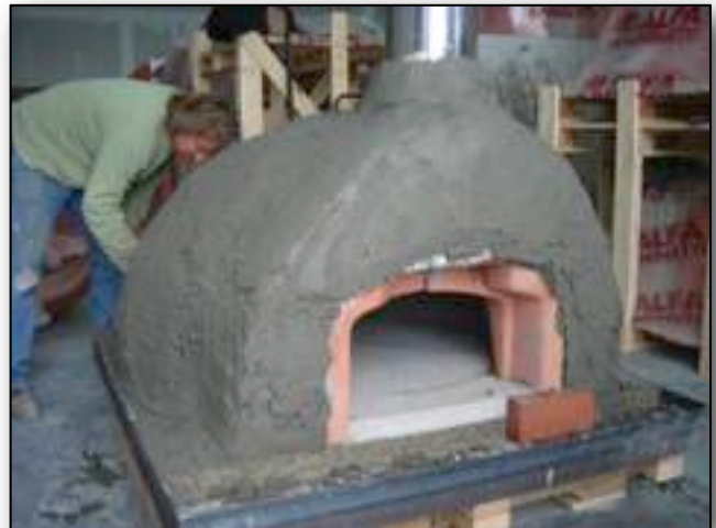
10.3 Rough coat of stucco on wire lathe.
