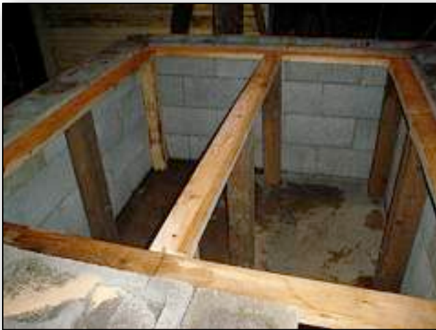
3.1. The form bottom ready for the Hardibacker.
