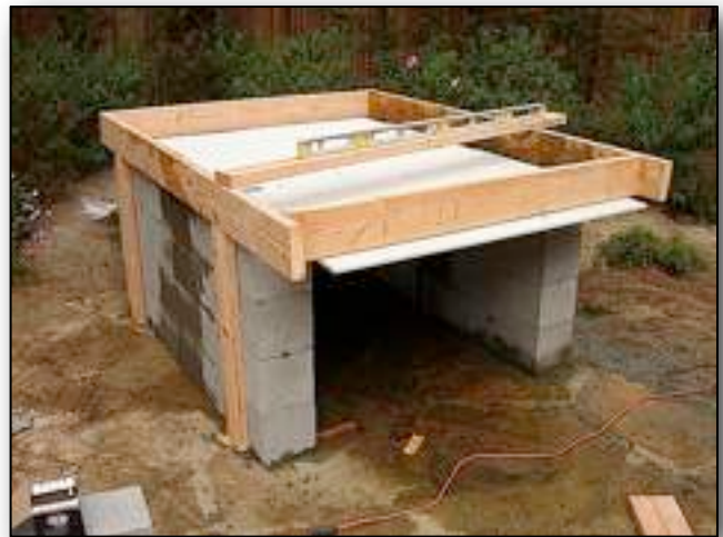
3.3. Hardibacker and form set in place.
