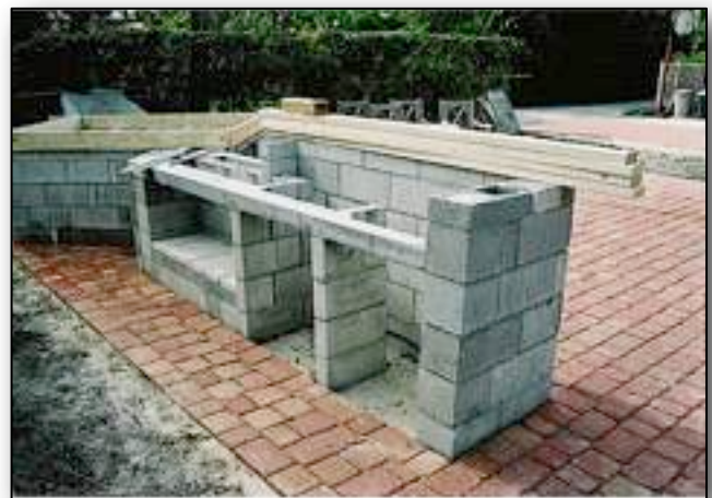
2.6. Stand with cast lintels.
