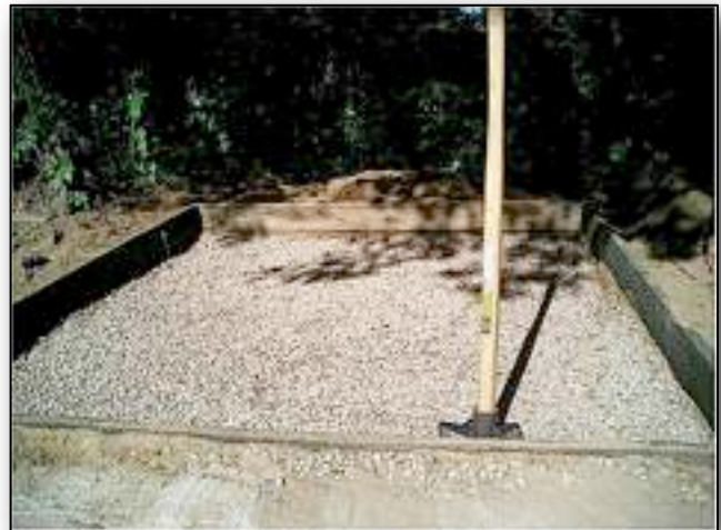
1.2. A gravel or crushed rock bed.
