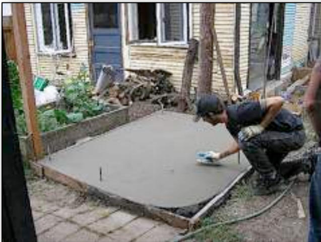
1.4. The finished foundation ready to cure.
