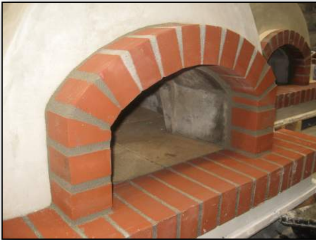
8.1 The Giardino brick arch on a brick oven landing.
