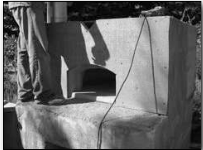
11.4. Attach concrete board.
