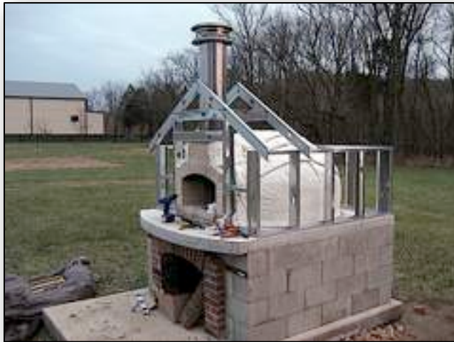
11.3. Metal studs and a gabled roof.
