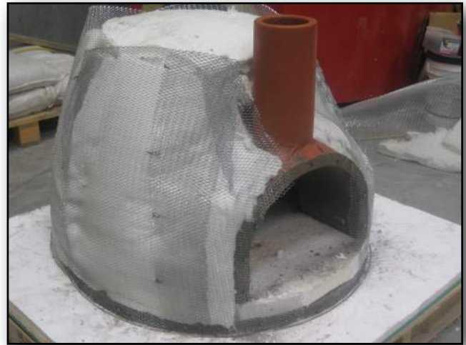
7.2. Stucco lathe holds the FB Board in place and can shape the Igloo.
