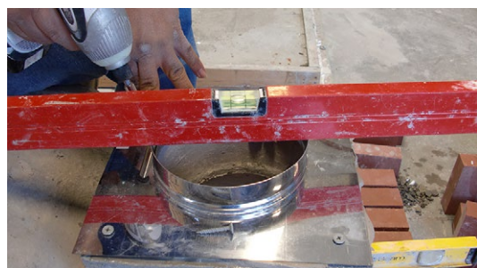
6.6. Check for level.
