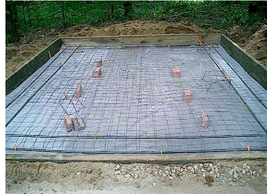
1.1. Framed, lined, with wire mesh and rebar.
