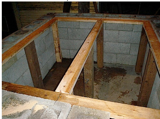
3.1. The form bottom ready for the Hardibacker.
