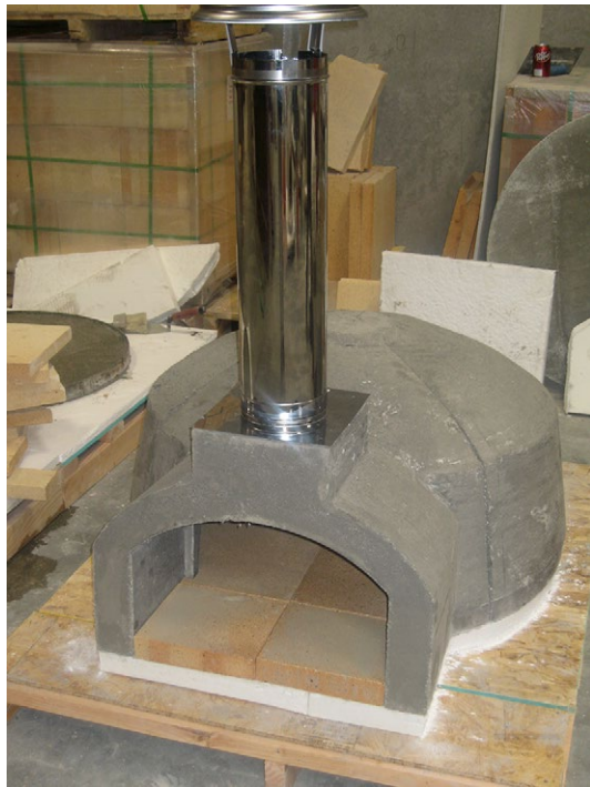
6.1 Casa2G with single wall stainless steel chimney.
