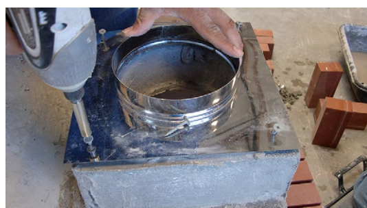
6.5. Screw the anchor plate in place.
