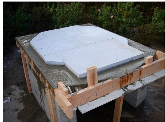
3.6 FB Board set in place.
