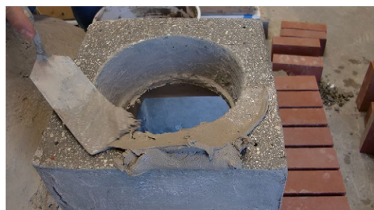
6.4. Apply a bead of refractory mortar.
