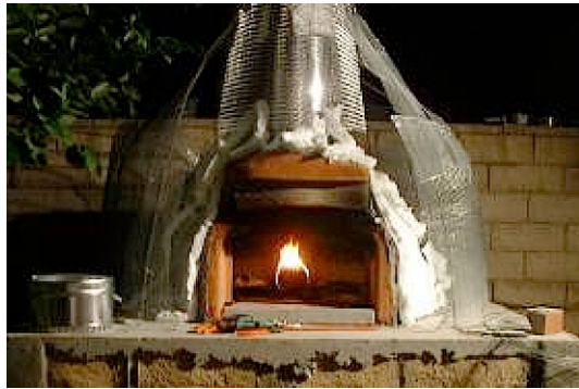
9.1 Rebar and lathe shape the Igloo.
