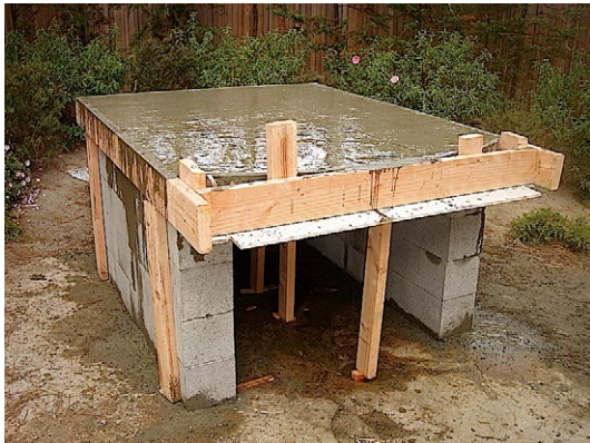
3.5 Structural layer waiting on insulating layer.
