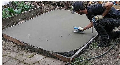
1.2. The finished foundation ready to cure.
