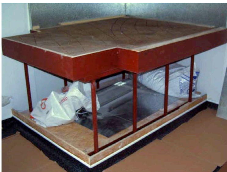
Installed Forno Bravo prefabricated stand and insulated oven base for a Ristorante 110 oven
