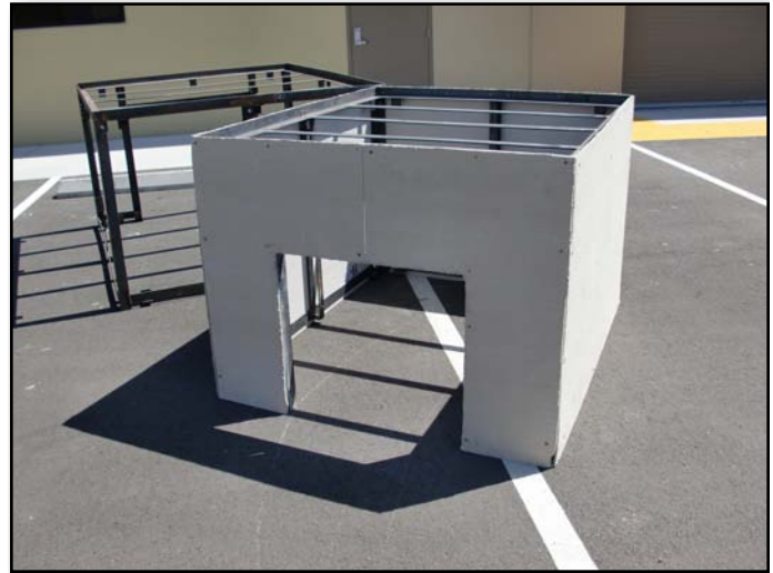
Pre-cut and pre-drilled backer board panels.
